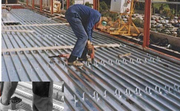
Application of Hilti shear connectors
