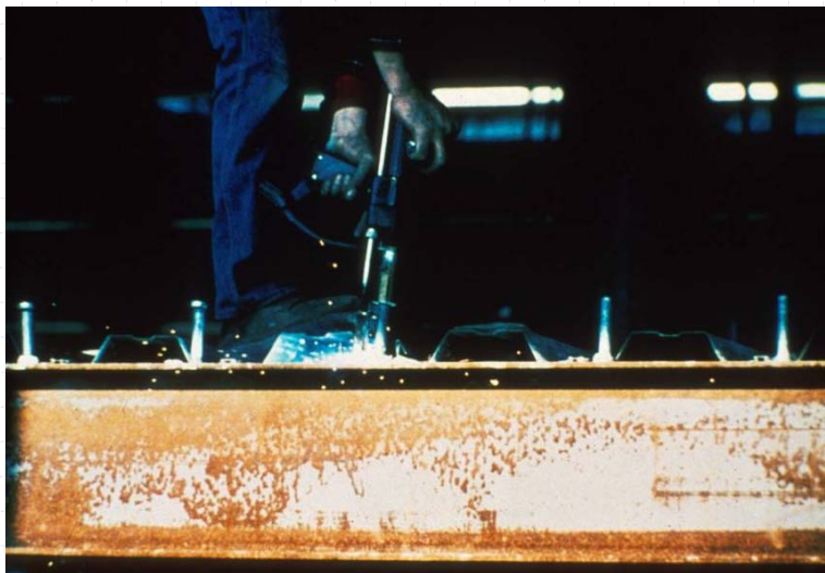
Semi-automatic welding of the shear studs
