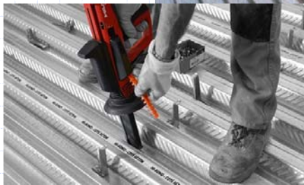
Application of Hilti shear connectors
